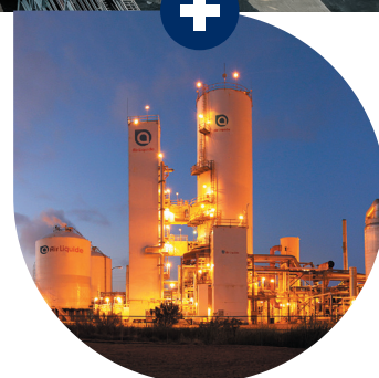
Air Separation Unit
