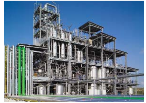
PHOTO: AIR LIQUIDE ENGINEERING & CONSTRUCTION
