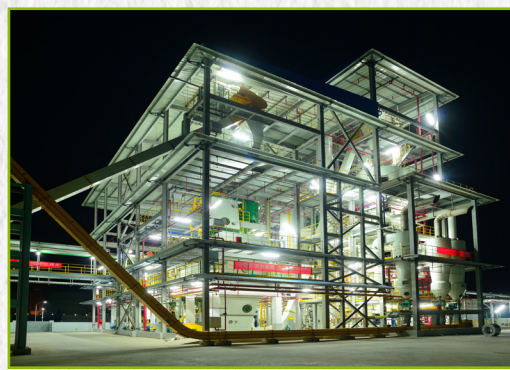
Lurgi Sliding Cell Extractor – Mega Oilseed Complex, China
