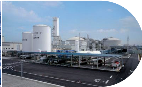
Hydroedge - Air Liquide Air Separation Unit integrated in LNG terminal (only daily start&stop shift)
