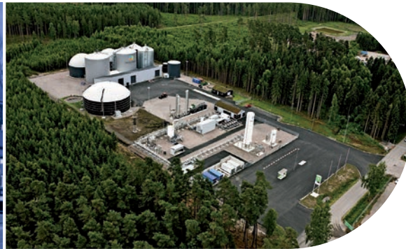
Air Liquide operates 10 biomethane production units in the world, incl. the Bio-LNG plant in Lidköping, Sweden
