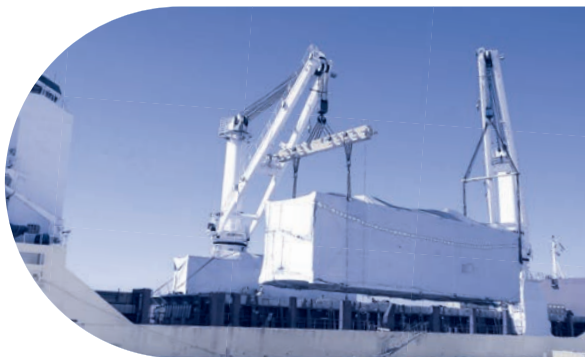
Air Liquide mid-scale (0.66 Mta) LNG project under construction in Europe
